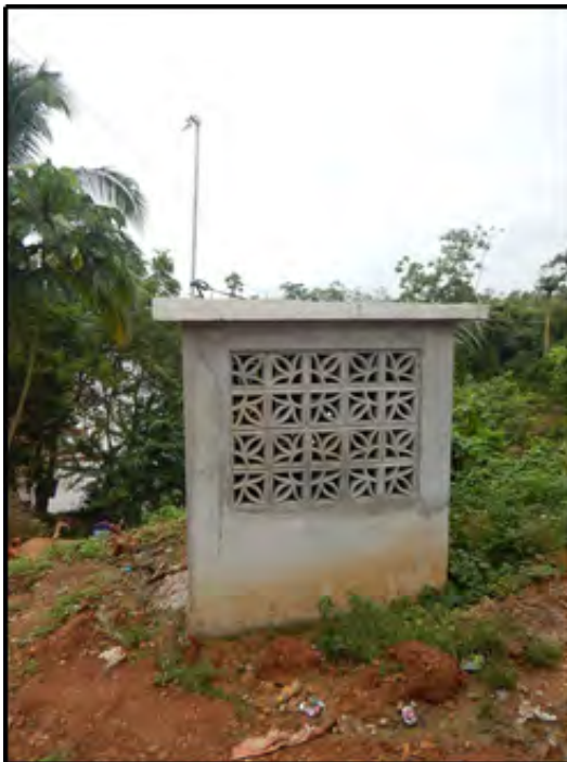
Figure 10. Electrical control booth [1]
