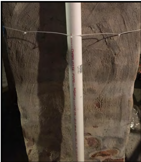
Figure 38. branch line attachment to concrete structures using zip ties [1]
