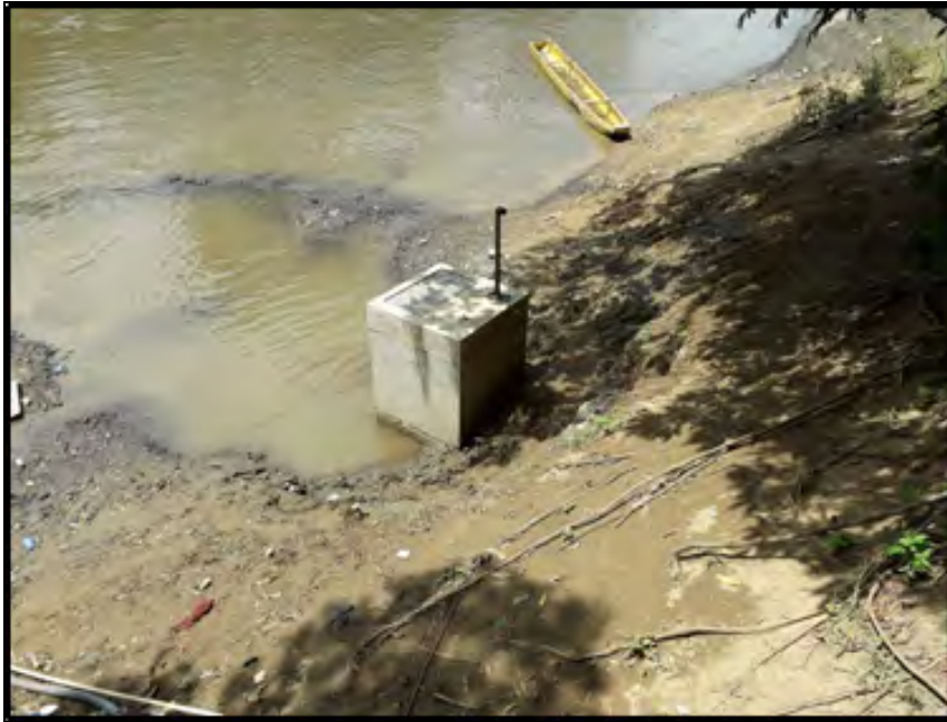
Figure 9. Existing intake structure in the Chucunaque River [1]
