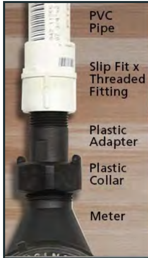
Figure 36. Recommended water meter connection [15]
