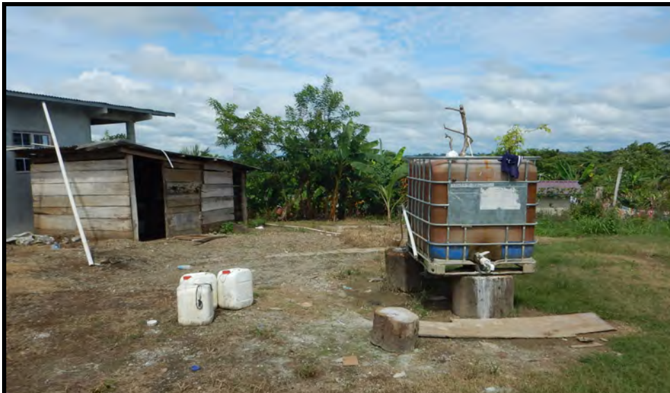
Figure 5. Independent water system pumps from Chucunaque River to residence [1]
