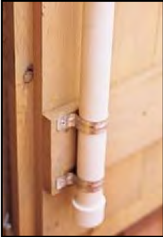
Figure 37. branch line attachment to wooden structures using metal pipe strap and nails [16]
